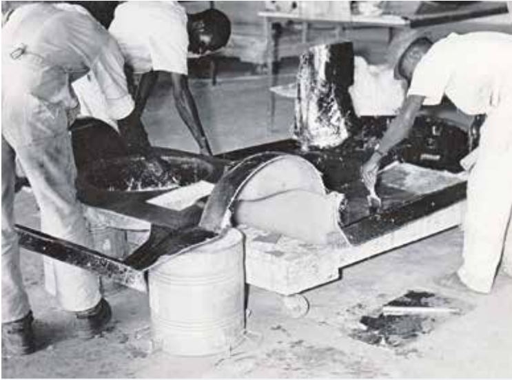
Floor pan construction.
