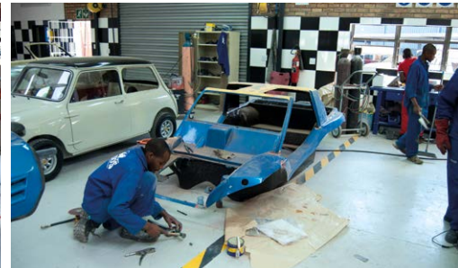
Beach buggies are hot with collectors at the moment and this one needs lots of work on the fibreglass body before a paint can be shot. Preparation is the key to a good fibreglass finish.
