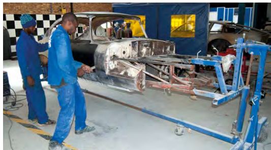
After hours of cutting out the rot, even more hours cutting and shaping new metal to fit, this Jaguar E-Type is starting to look like the iconic sportscar we all know and love. It's had sills, floors and a myriad of other panels worked on
