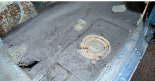
While the BMW 3.0CSL was in reasonable all round shape the floorpan was not. This meant cutting out all the rot and fabricating new ones from scratch. A lot of time and effort went into putting in the correct reinforcements to indentations.
