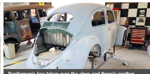
Beetlemania has taken over the shop and there's another early one nearing the paint-worthy stage. This oval window took a fair amount of fabrication to fix rotten panels. The rear valence for example was made up from scratch. Once painted the client will take the body away and complete the build.
