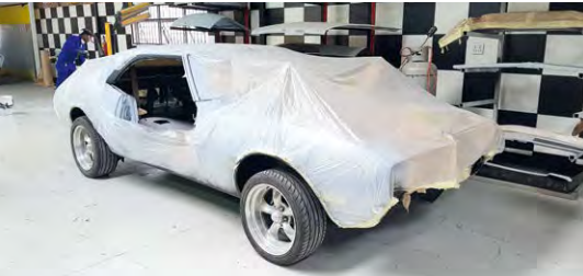
As mentioned before, this Camaro drove into the shop but suffered serious gremlins under the paintwork. Botched jobs were numerous but have been sorted now by cutting and removing the issues and replacing with fresh metal. It is ready to paint.
