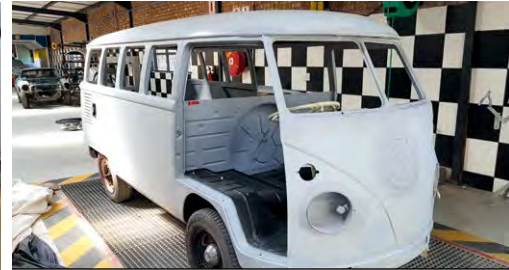
Remember the red splittie that looked reasonable on entry to the shop? Well, it wasn’t. Under the paint we found heaps of filler and even more fibreglass patchwork. We stripped it to bare metal, removed the botched work and made up new metal parts and panels to suit. It’s now finally ready for paint and will be done in a two-tone white/blue hue before Generation Old School assemble.
